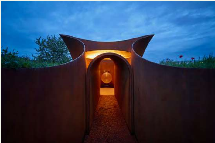
The 2200K illumination resonates with the warmth of Corten steel, casting a soft amber hue that soothes the night-adapted eye. These ribbons of light provide legibility without distraction, allowing one to turn inward through this journey. Photo credit: Julien Lanoo
