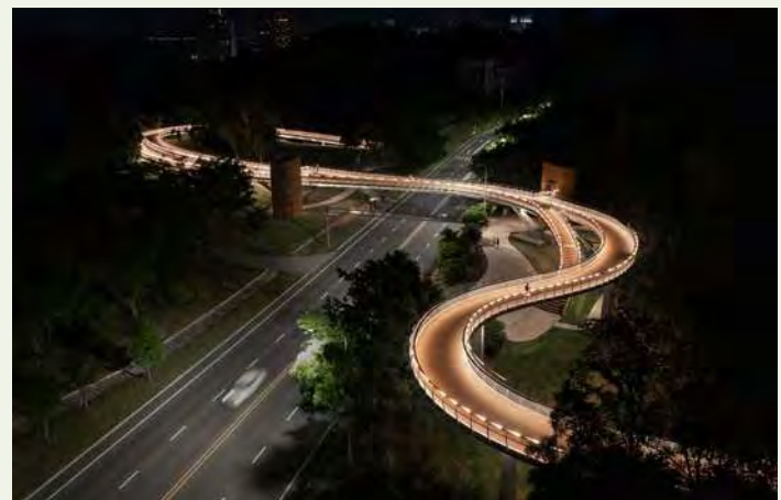
Zhuhai Banzhang Mountain Footbridge
